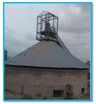
Covered clinker stock pile for storage of clinker with bag filter
