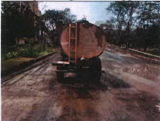
Water sprinkling for dust suppression (Annexure-7)
