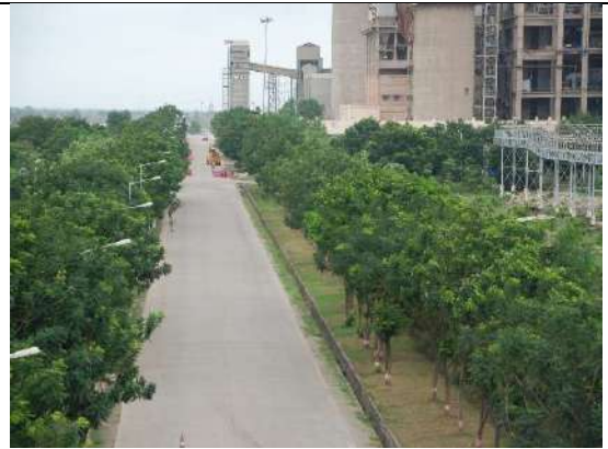
Description: Plant Internal CC Roads
