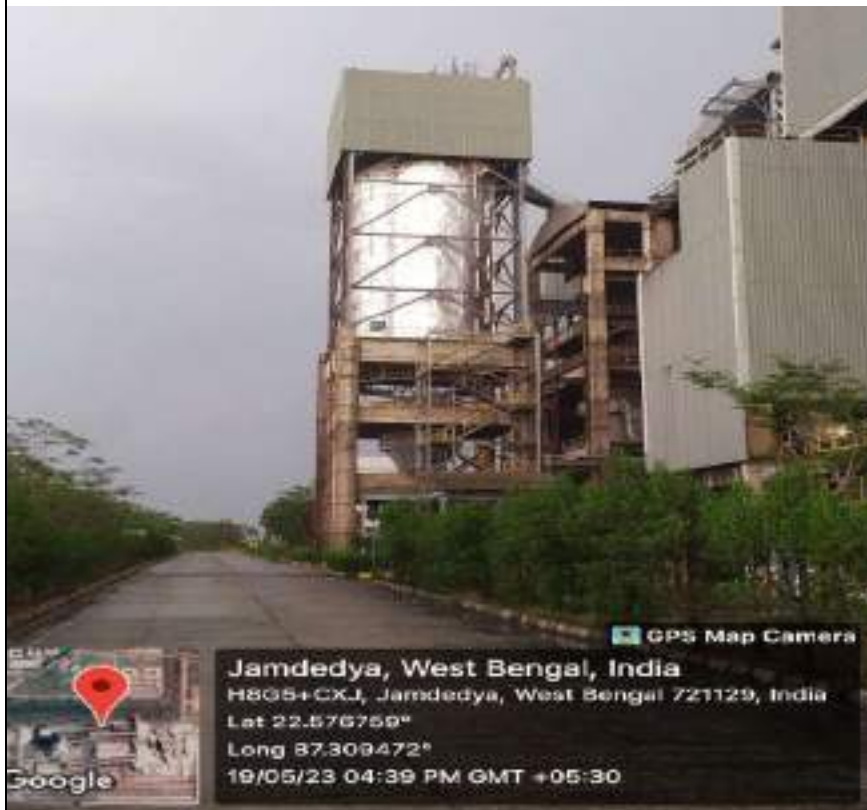
Covered Storage Bins (Photograph - VI)
