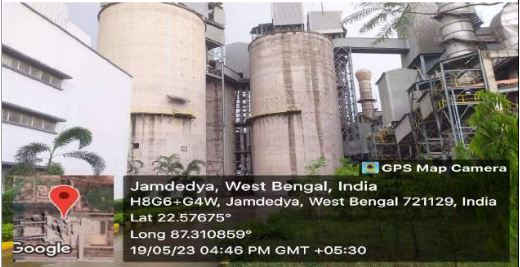
Closed Storage Silos with APCD(Photograph - IV)
