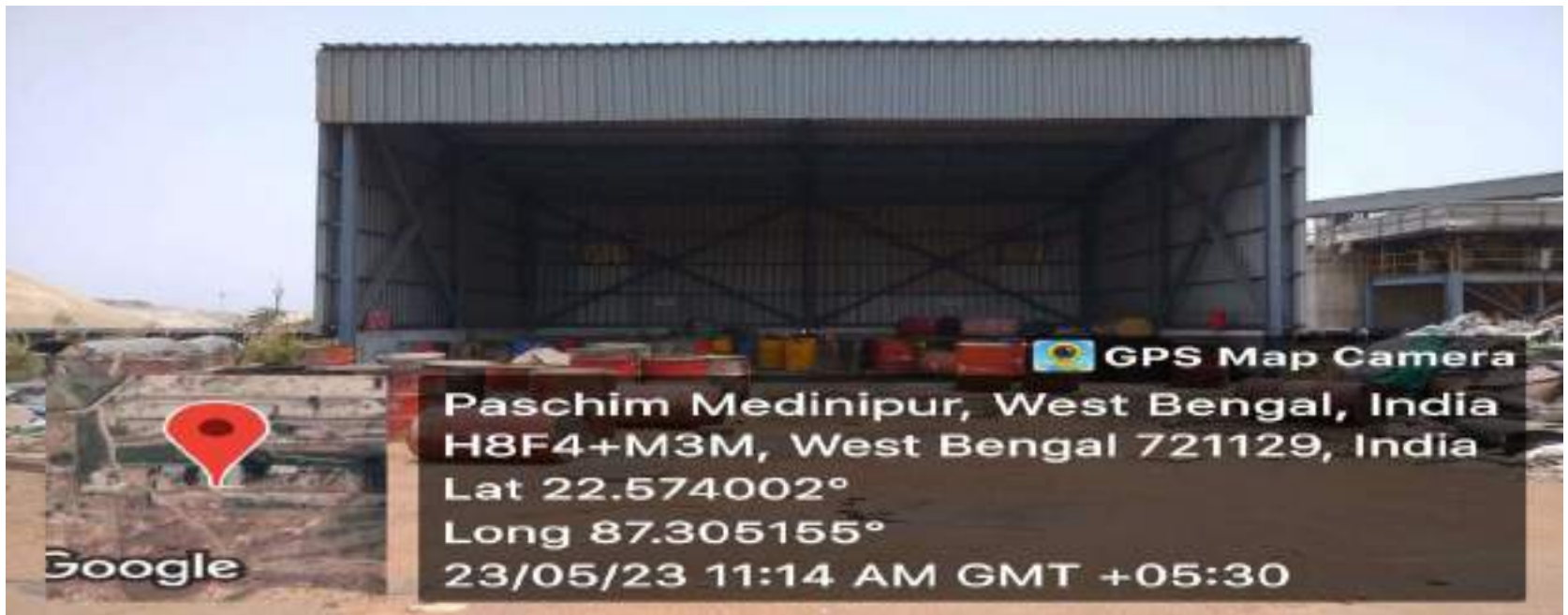
Hazardous waste storage facility inside the plant (Photograph - XVIII)
