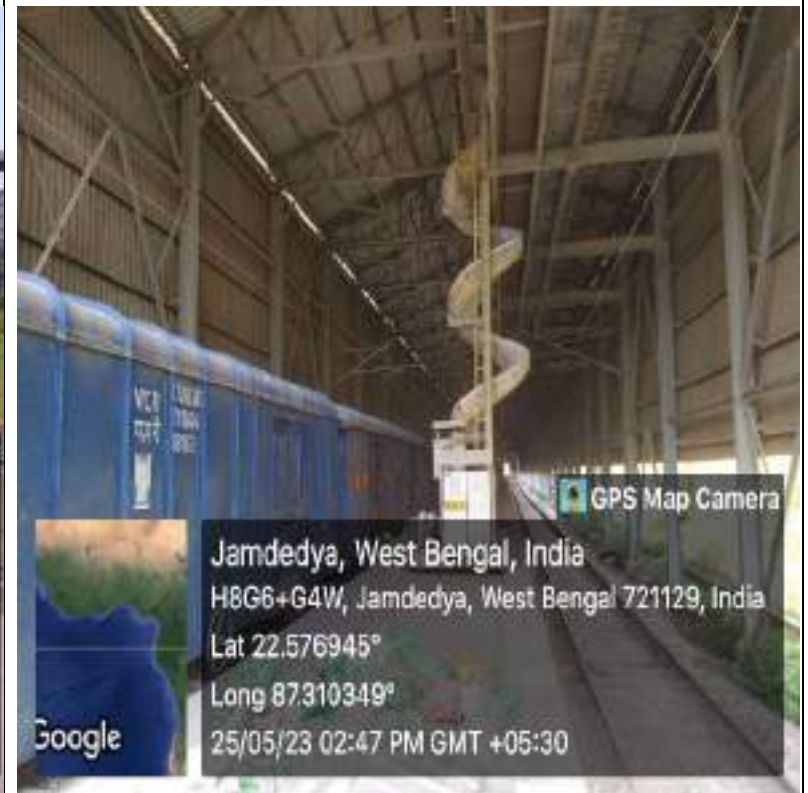
Covered Wagon Loading Area (Photograph-XII)
