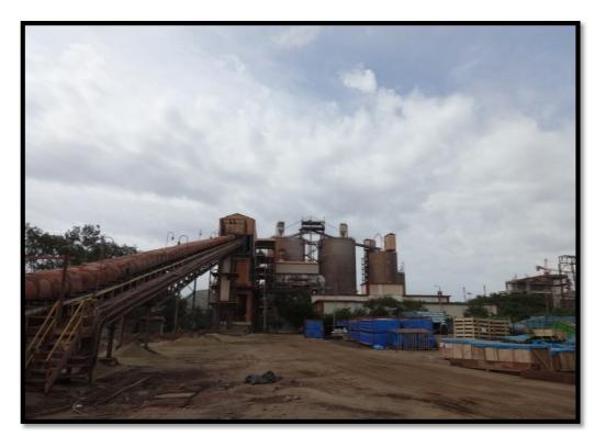
Covered belt conveyer, silo with bag filter for the storage of cement &GGBS
