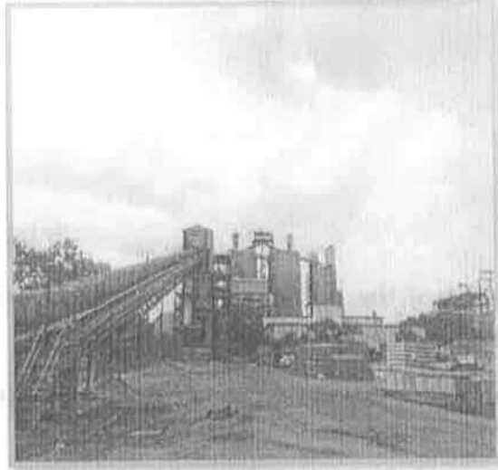
Bag filters provided at raw material transfer point with covered beld conveyer
