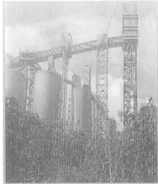
Silo provided for storage of product along with bag filter
