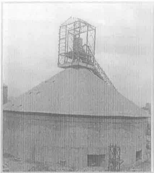
Covered clinker stock pile for storage of clinker with bag filter
