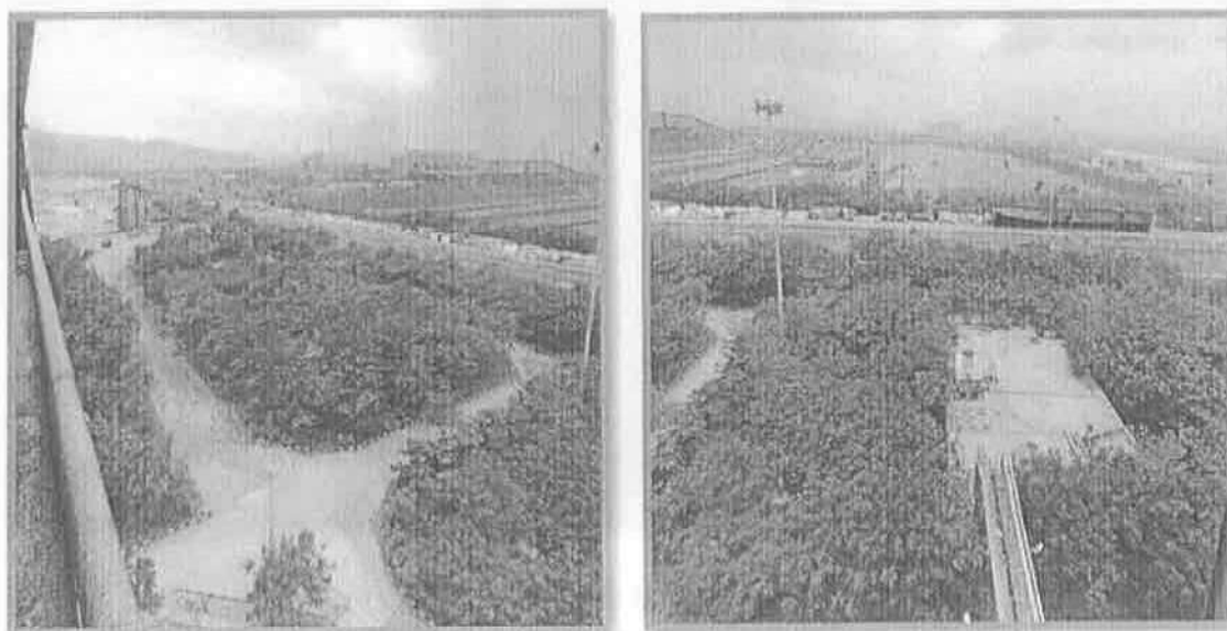
Green belt development inside the plant area
