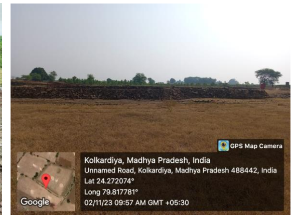
Bund along-with Mine Pit
