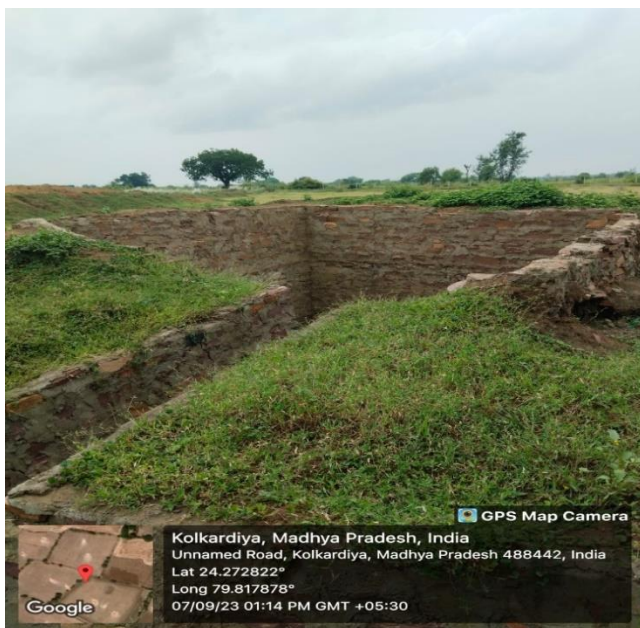
Siltation Pit -1 (L&W 5.3 and Depth 4.3 meter)
