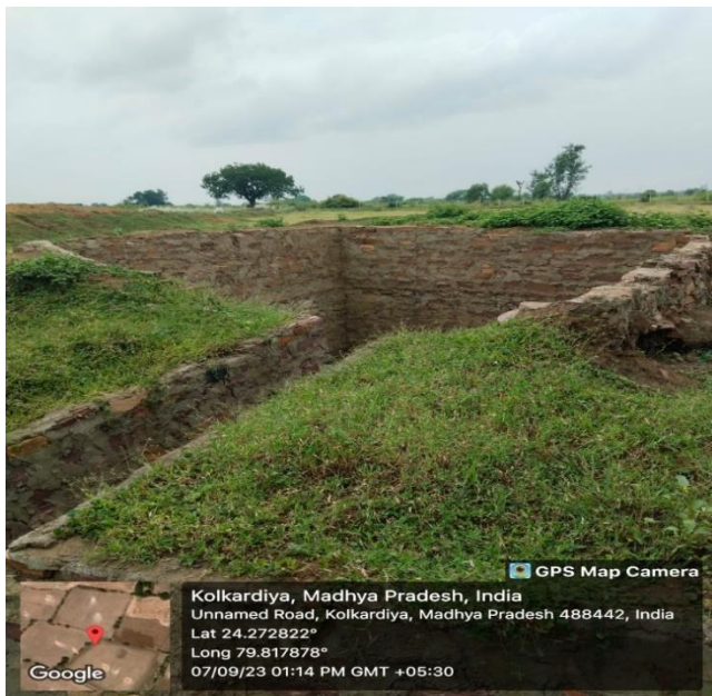
Siltation Pit -1 (L&W 5.3 and Depth 4.3 meter)
