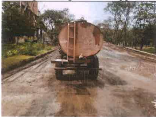
Water sprinkling for dust suppression (Annexure-7)
