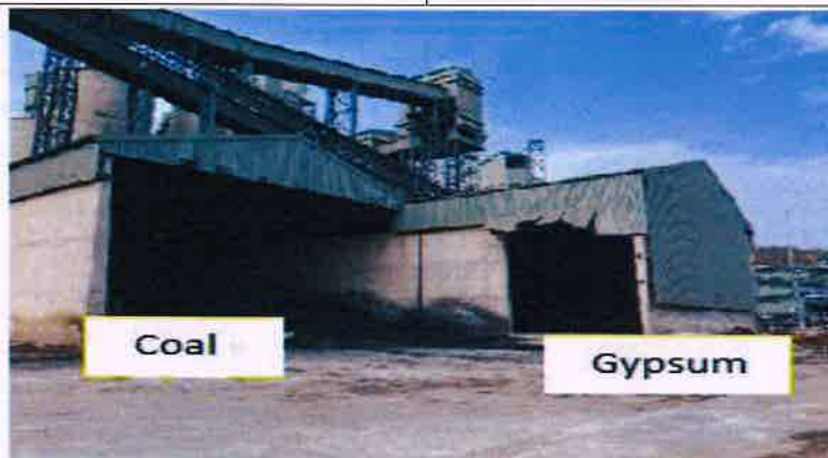
Covered Shed for Raw Material Storage
