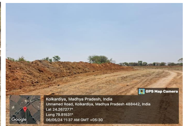
Bund along-with Mine Pit
