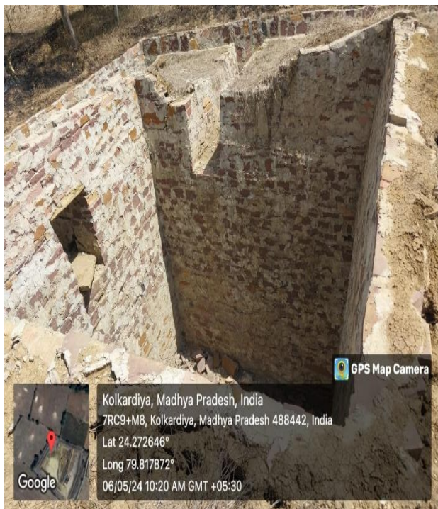
Siltation Pit -1 (L&W 5.3 and Depth 4.3 meter)
