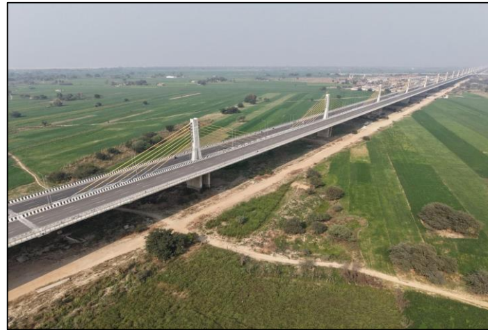
L&T Daewoo- Patna Bridge
